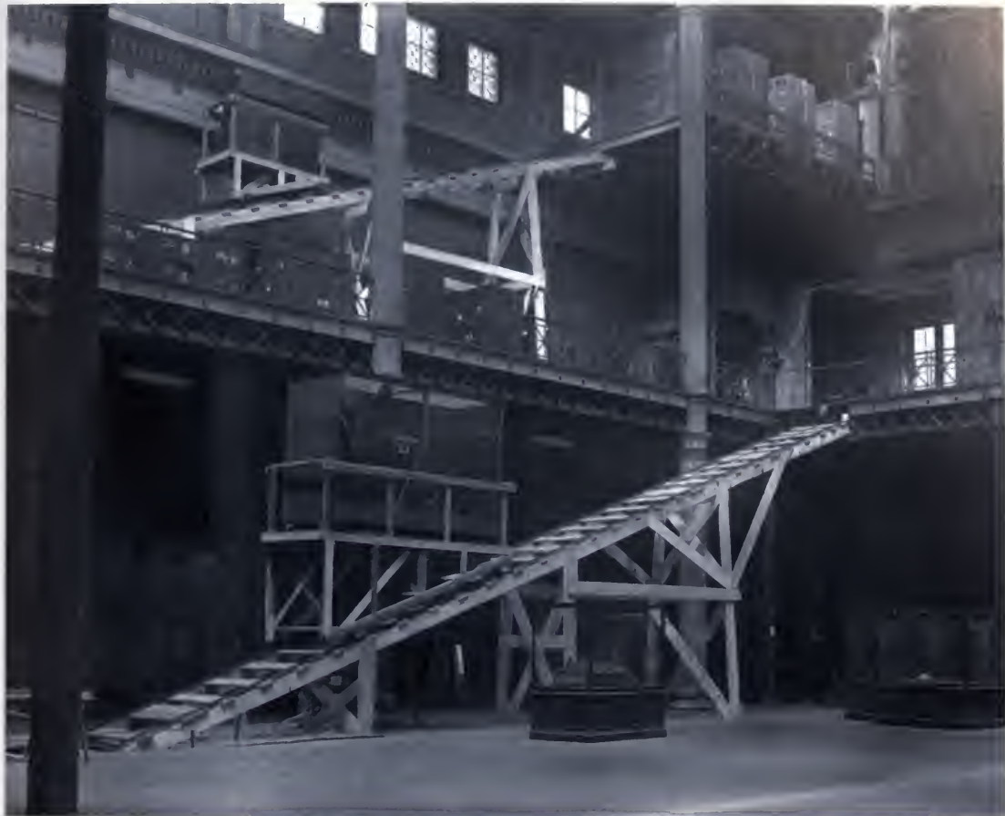
FIG. 16.1. Field Columbian Museum exhibits in Jackson Park being moved to the new Field Museum building in Grant Park.
